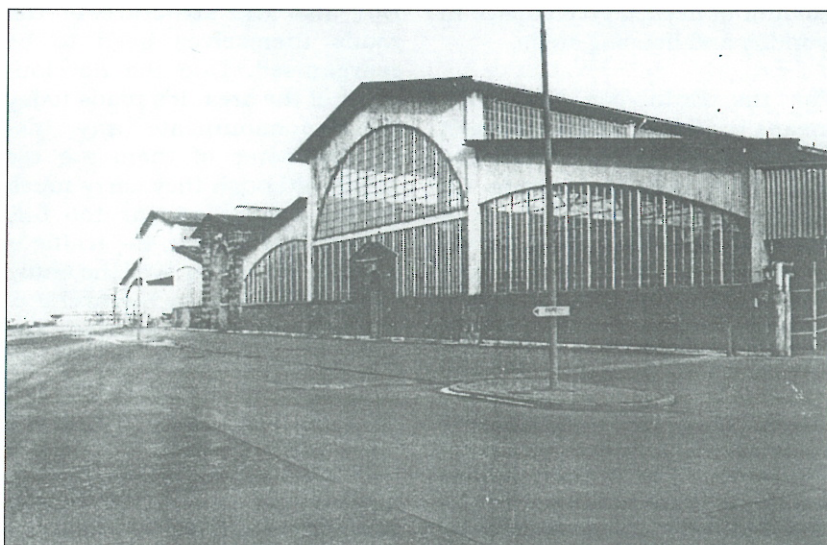
Picture 5: After the removal of the Slaughterhouse, the protected Cattle-Hall and 25 surrounding hectares are left unused
