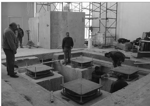
Figure 2: Installation of seismic isolation for the statue of Hermes at the Olympia museum (source: Koumouisis, 2007).
