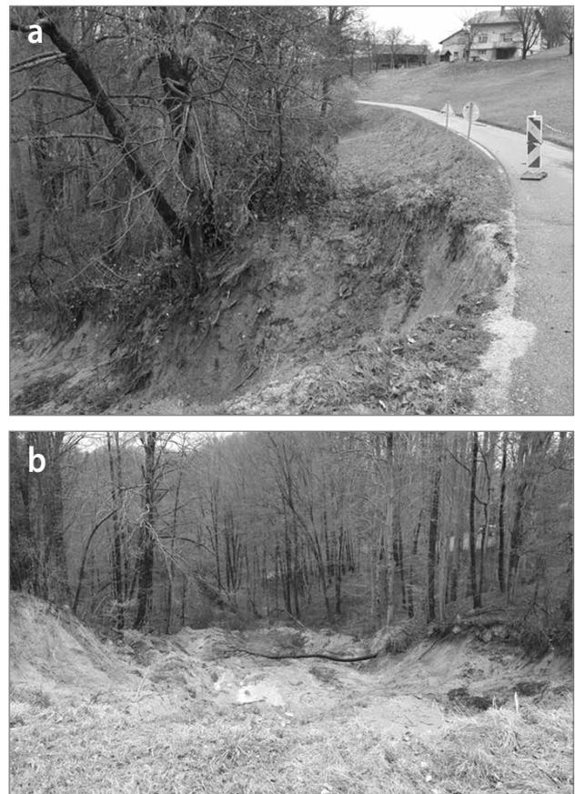
Figure 2: a) typical slope failure resulting from water infiltration into the slope and simultaneous runoff of stormwater from the road, and b) the body of the landslide with earth ridges at the base of the slope (photo: Bojan Žlender).
