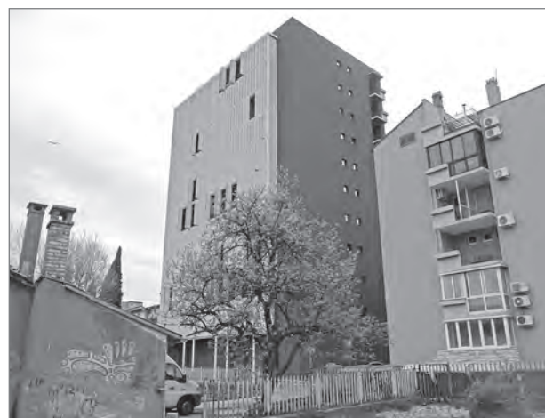
Figure 2: View of the renovated Tomos Tower Block from the courtyard of the Tutto ex Gavardo Palace (photo: Tina Cotič).
