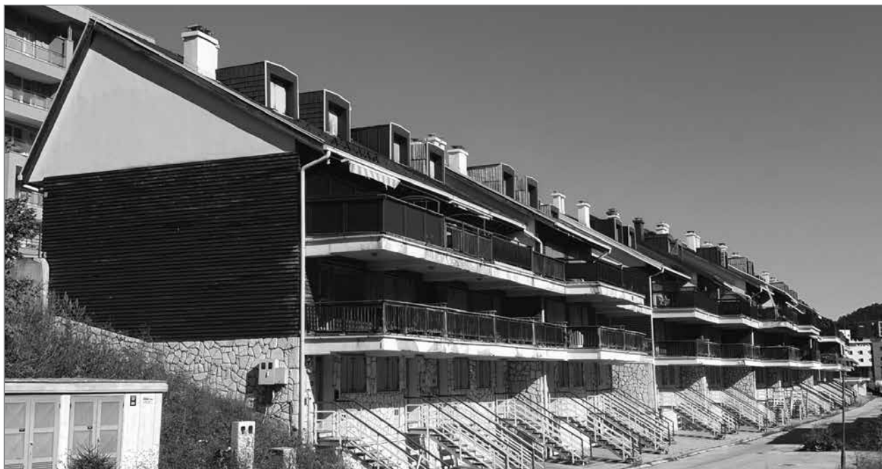
Figure 13: The first accommodation built at Babin Do, Izet Arslanagić, 2005 (photo: Alma Hudović Kljuno).
